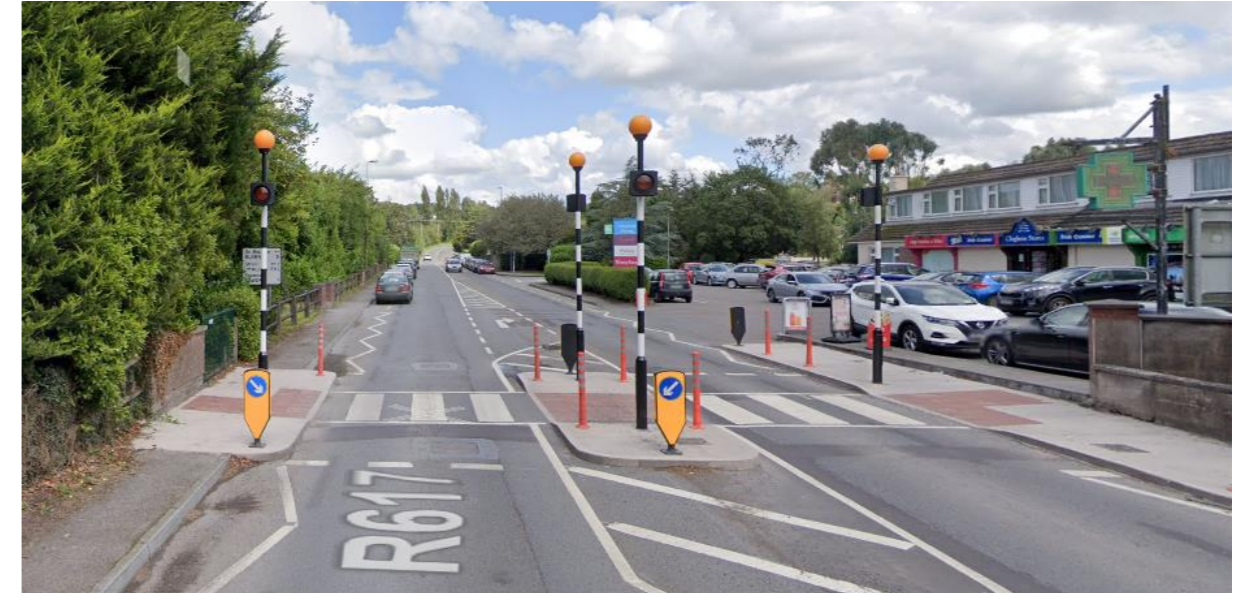
Fig 11.1: Existing Zebra Crossing on the R617
